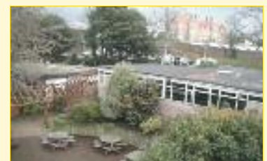
Bird's eye view of the site for the class room block
